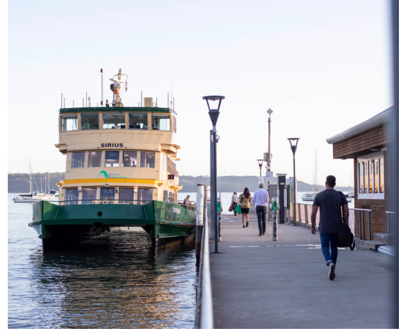
Double Bay Wharf
